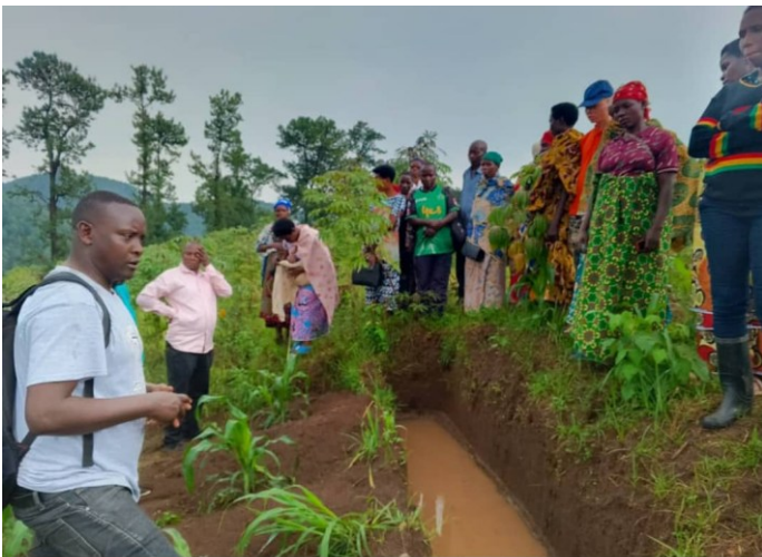
Field visit by partners and beneficiaries to the site where contour lines are being laid out on Bugume hill.
